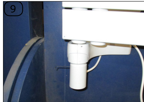
ELECTRICAL APPLIANCE ONLY: Loosen the head with a 1.5 hex key. Extract the head, the heating element power cable should come with it.
