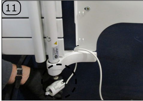
ELECTRICAL APPLIANCE ONLY: Cut the power cable from the heating element so you can extract it from the wall mounting. The blower can now be completely removed.
