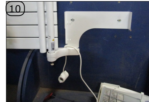
ELECTRICAL APPLIANCE ONLY: Loosen the head with a 1.5 hex key. Extract the head, the heating element power cable should come with it.
